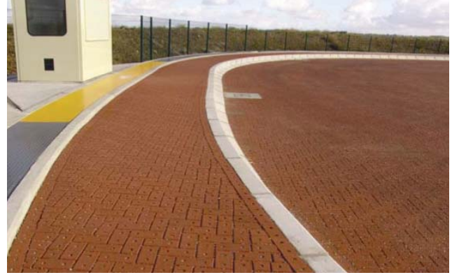
Photo 2 Permeable Clay Pavement
