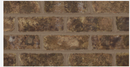
Identical brick sample panels incorporating different mortar colors.
